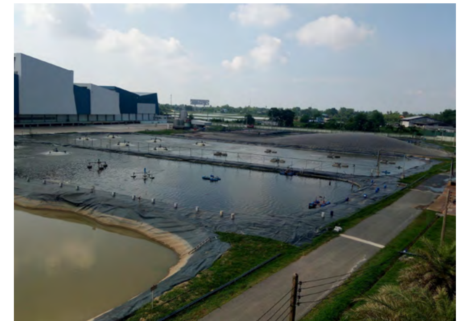
Wastewater treatment plant at Dairy Plus, Thailand
